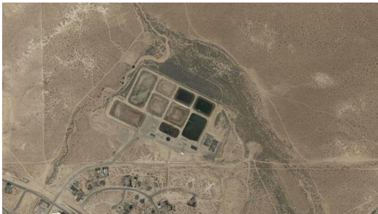
Figure 4-1 City of California City's WWTP (2023)
