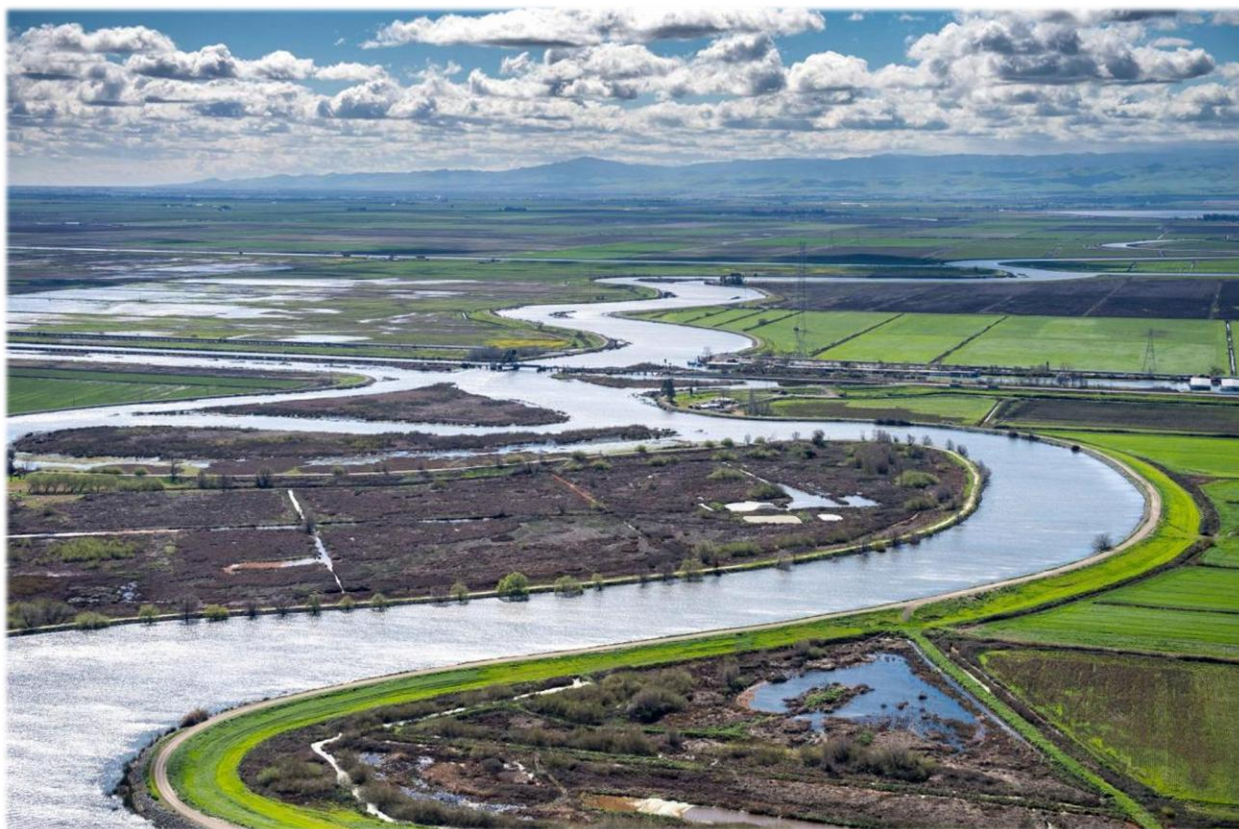
Figure 3-5 State Water Project
