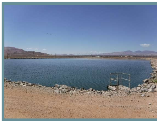
MPUD's wastewater percolation ponds
