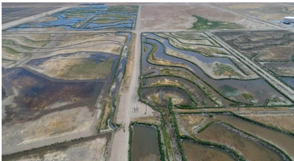
Figure 3-1 AVEK's Westside Water Bank
