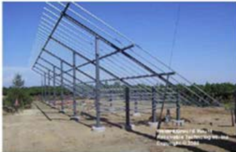
Typical Fixed-Tilt Mounting Structure
