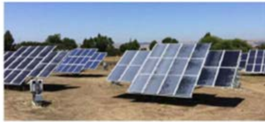
Typical Dual-Axis Tracking Solar Panels
