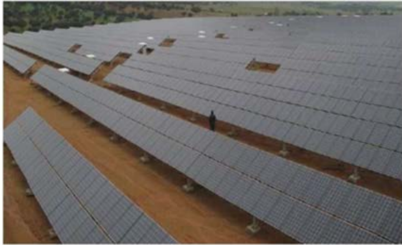
Typical Fixed-Tilt Solar Panel Rows
