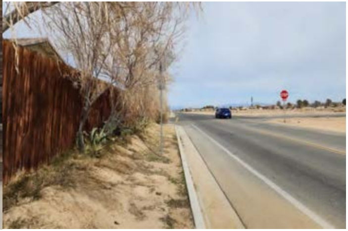
AFTER looking North
