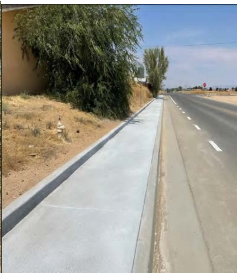
AFTER looking North
