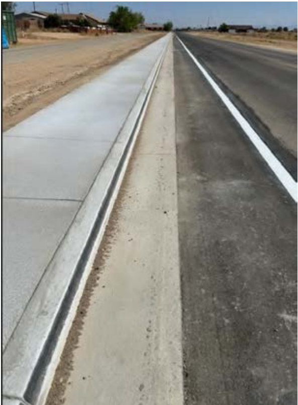
AFTER looking North
