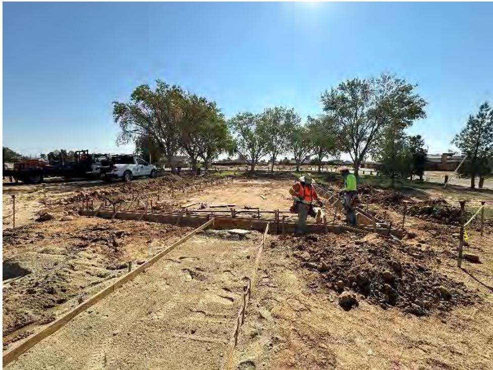
Looking North-East during construction of playground
