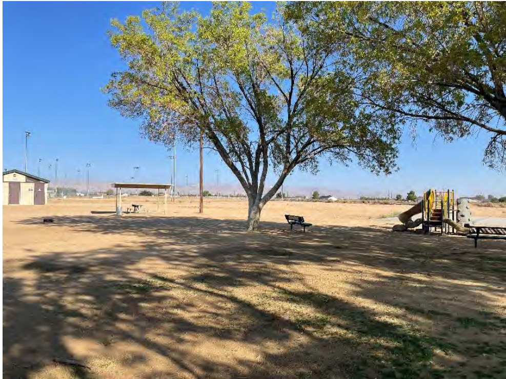
Looking North during construction
